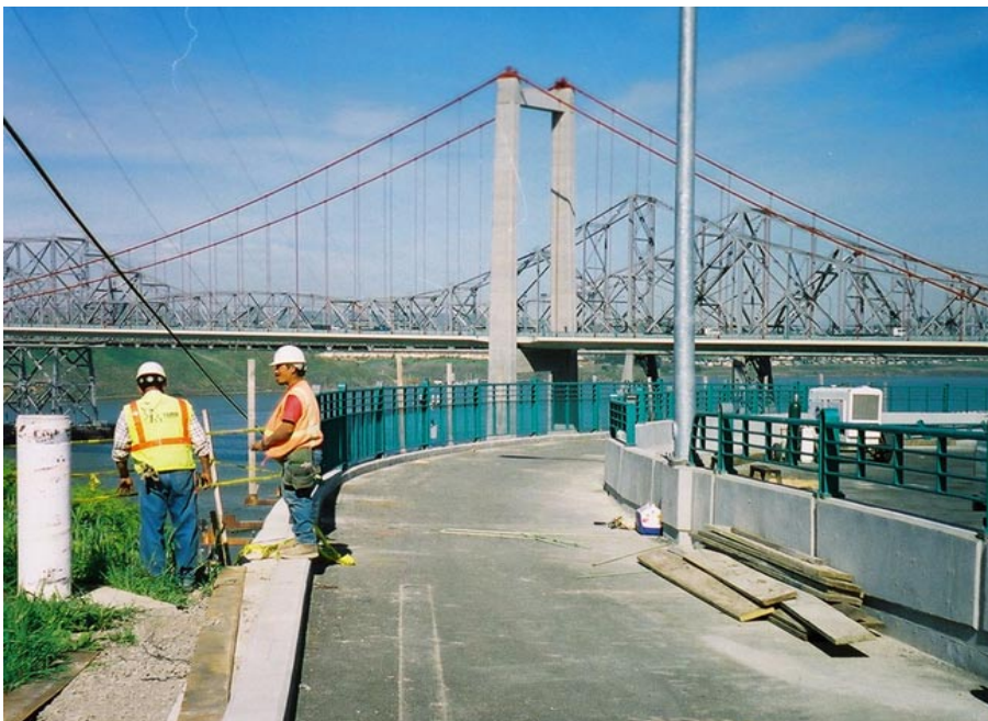
Construction progress on the Zampa bridge path.
